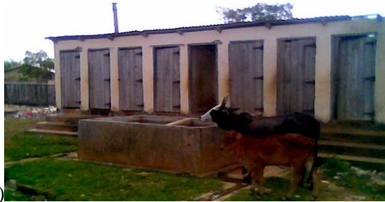
(Welfare Centre Toilets)
